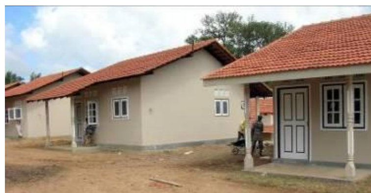
House Reconstruction, Galle (Sri Lanka )
